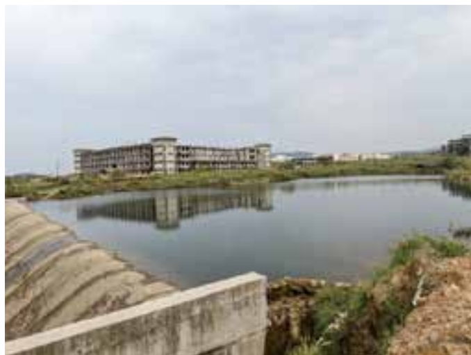
WATER STORAGE RESERVOIR
