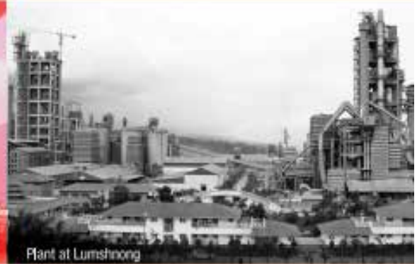
Plant at Lumshnong
